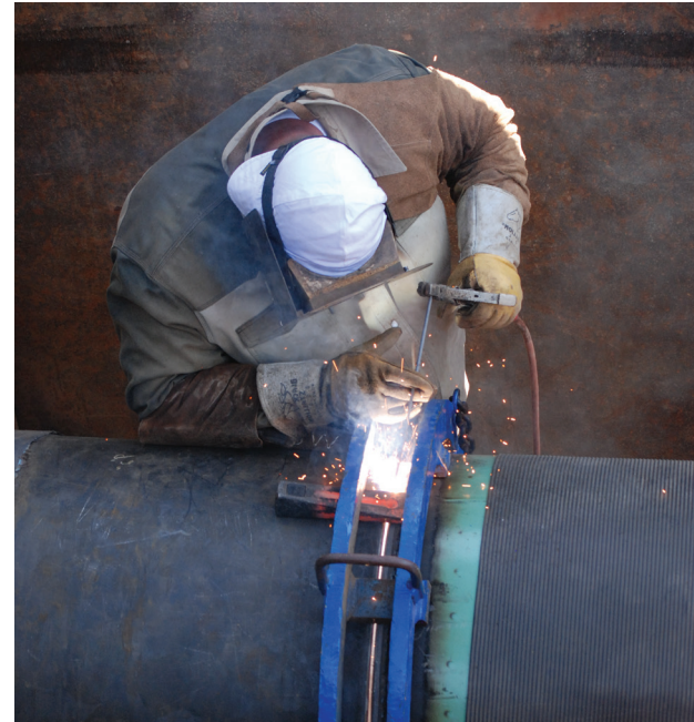
A pipeline test head cap is carefully welded to the end of a pipeline segment to be pressure tested.
