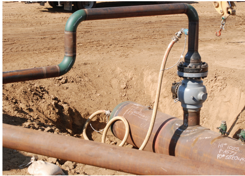
Water is pumped into a test head to conduct a pressure test.
