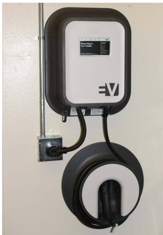
Figure A.3-1: Level 2 EV Charging Unit
