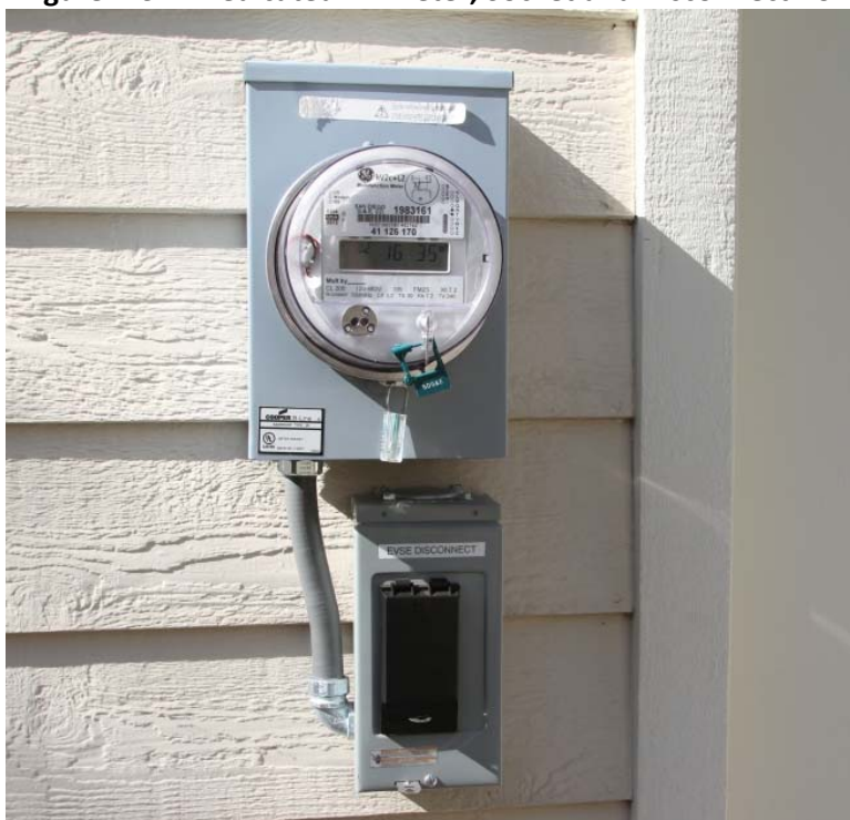
Figure A.3-2: Dedicated EV Meter, Socket and Disconnect Box
