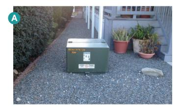
A-B: A single-phase transformer is typically housed in a green box and mounted on a concrete pad, like the equipment shown here. Clearances must be maintained for access: at least 8 feet in front of the door and 18 inches on the other three sides. Although such equipment is above ground, it's technically considered underground equipment because it's connected to underground electric lines, not overhead power lines.
