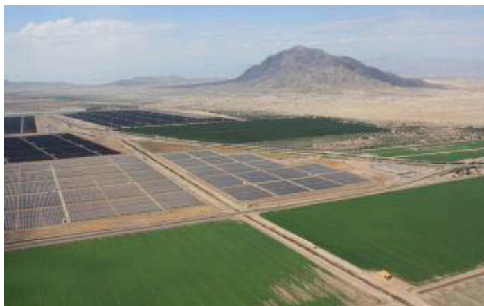
Figure 3 - Aerial view of Centinela Solar Energy and CSOLAR IC South facilities in Imperial Valley, CA
