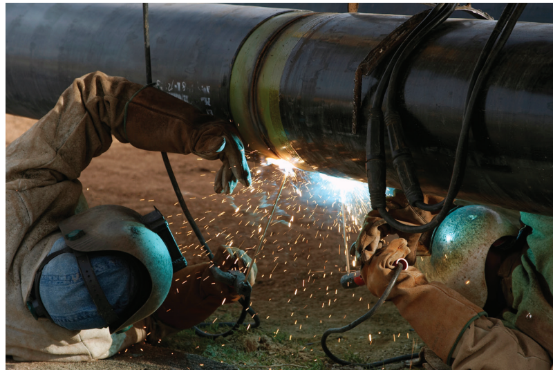
Workers carefully weld two pipeline sections together.
