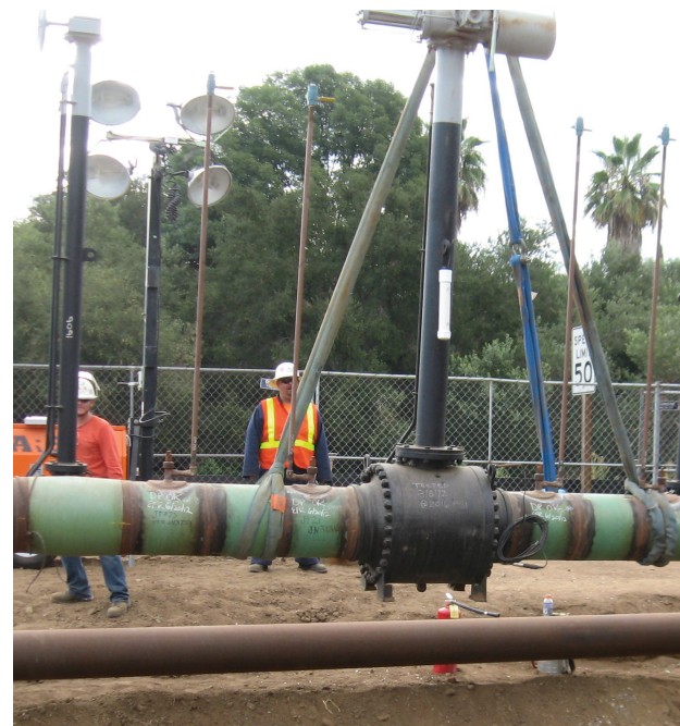
A valve in a pipeline section with an actuator on an extension stem in the process of being installed.
