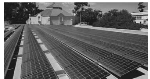
More than 30 local facilities, including the Reuben H. Fleet Science Center, host solar panels that contribute clean energy to the community.
